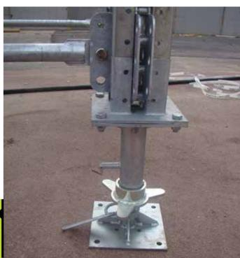
The fine adjustment of the vertical alignments of the shoring structure is carried out by means of highly-resistant levellers with a load capacity of 250 kN per vertical alignment.
